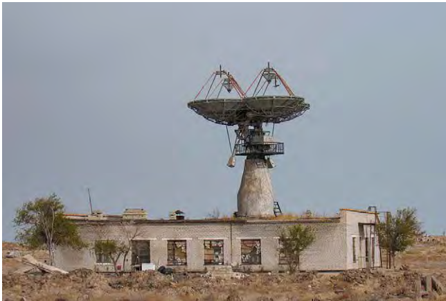
A dilapidated facility at Sary-Shagan (Credit: Nikolay Bulykin, cc-by-sa 4.0).
