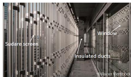
Photo 1. Sudare screen / maintenance deck
