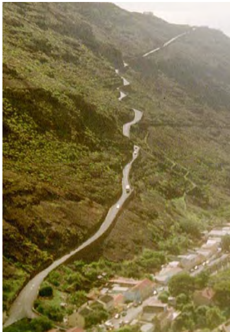
Figure 4.16: Ladder Hill Road out of Jamestown i
