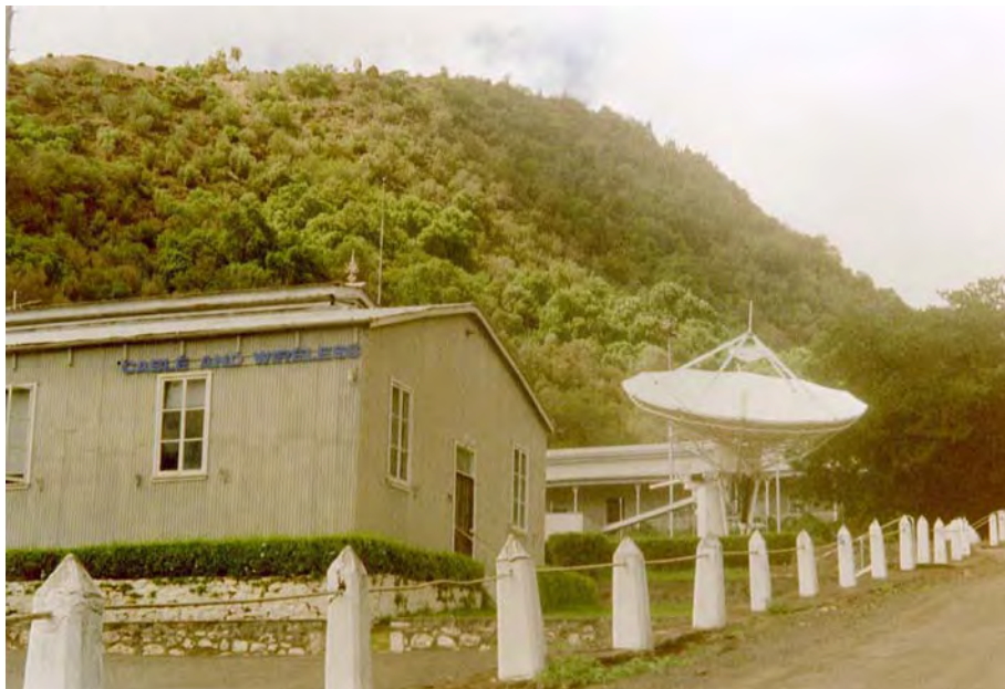
Figure 4.20: Cable and Wireless headquarters at the Briars i
