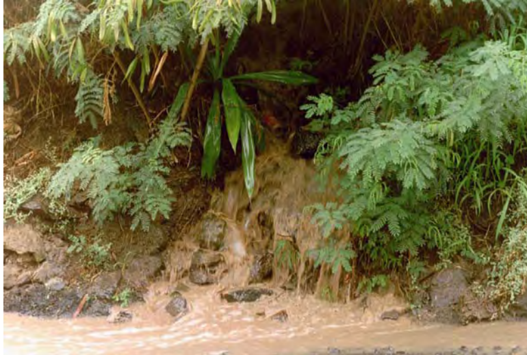
Figure 4.2: Erosion after a day of heavy rainfall i
