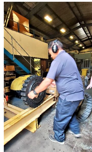
Merril preparing for installation of the new coupling on Generator No. 1
