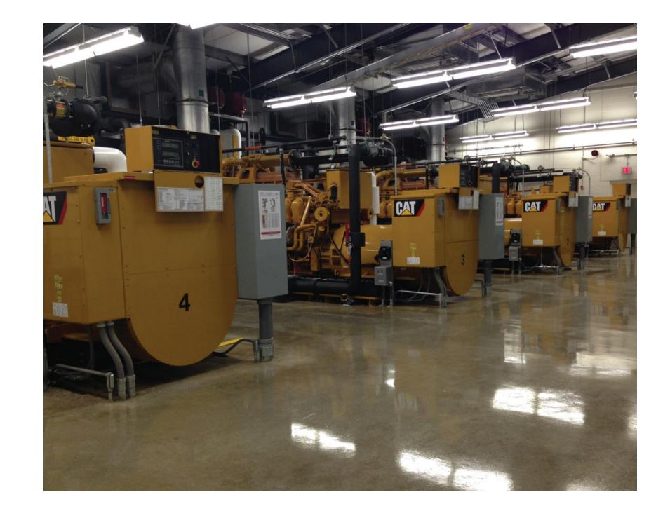
the site by transitioning from a large, traditional steam system to a Combined Heat and Power solution, harvesting heat from landfill gas powered generators through heat exchangers
