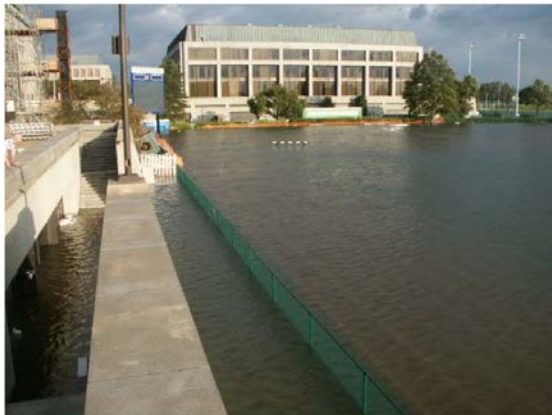
USNA academic buildings and athletic fields in aftermath of Hurricane Isabel ( http://www.naany.org/Hurricane_Isabel_strikes_USNA_2.htm )
