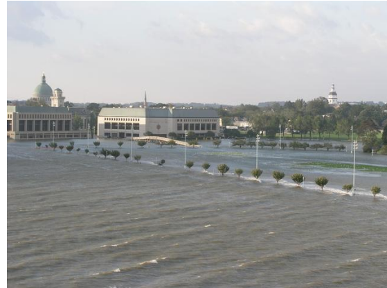
USNA flood damage due to storm surge ( http://icons.wunderground.com/data/wximagenew/a/awalex/0.jpg )
