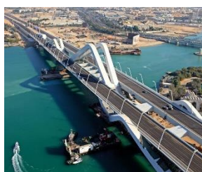
Sheikh Zayed bridge
