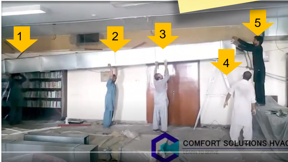
GI metal duct
