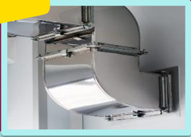
GI metal duct
