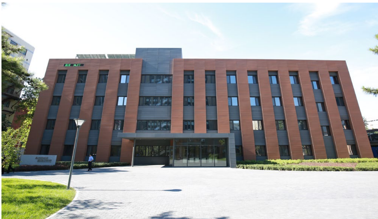
China Academy of Building Research
