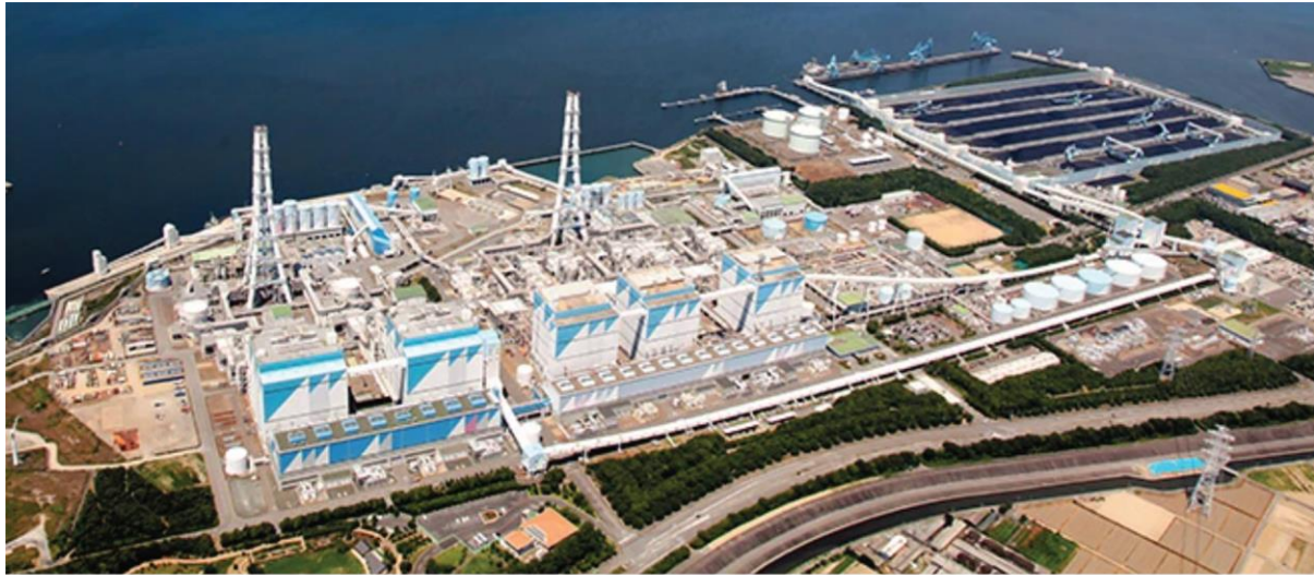
Figure 8 Hekinan coal-fired power plant (Shinden, 2021)
