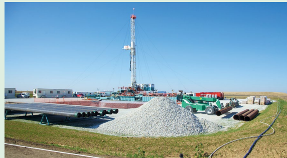
Figure 9. FutureGen Storage Site (Photo credit, FutureGen Alliance)
