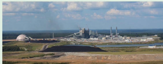
Figure 6. Kemper IGCC Power Plant (Mississippi Power, 2016)
