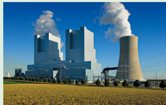
Figure 2. Neurath USC Power Plant (photo credit, RWE)
