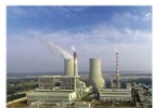
Shenhua Anqing Power Plant First Power Plant to Apply the 28MPa/600°C/620°C Steam Parameter
