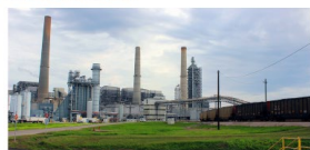
Carbon Capture Facility at Petra Nova
