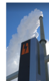
The Carbon Capture Test Facility located at the SaskPower Shand Power Station near Estevan, Saskatchewan
