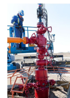
The Aquifer injector well during its installation
