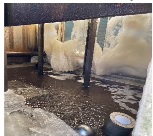
Freezing of common cooling towers Indirect Evaporative cooling towers
