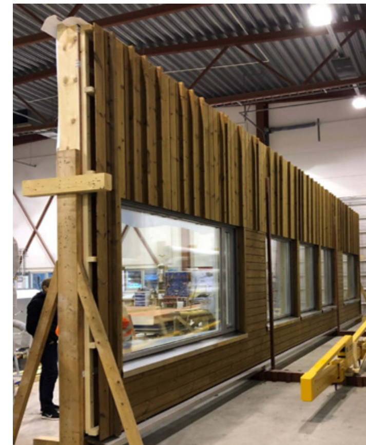
Very large format panels with integrated windows and cladding. An unconventional approach relying on tapes and gaskets is used to provide an interior finish and exterior wood cladding. (Mjøstårnet, The Tower of Lake Mjøsa – Moelven Limtre)
