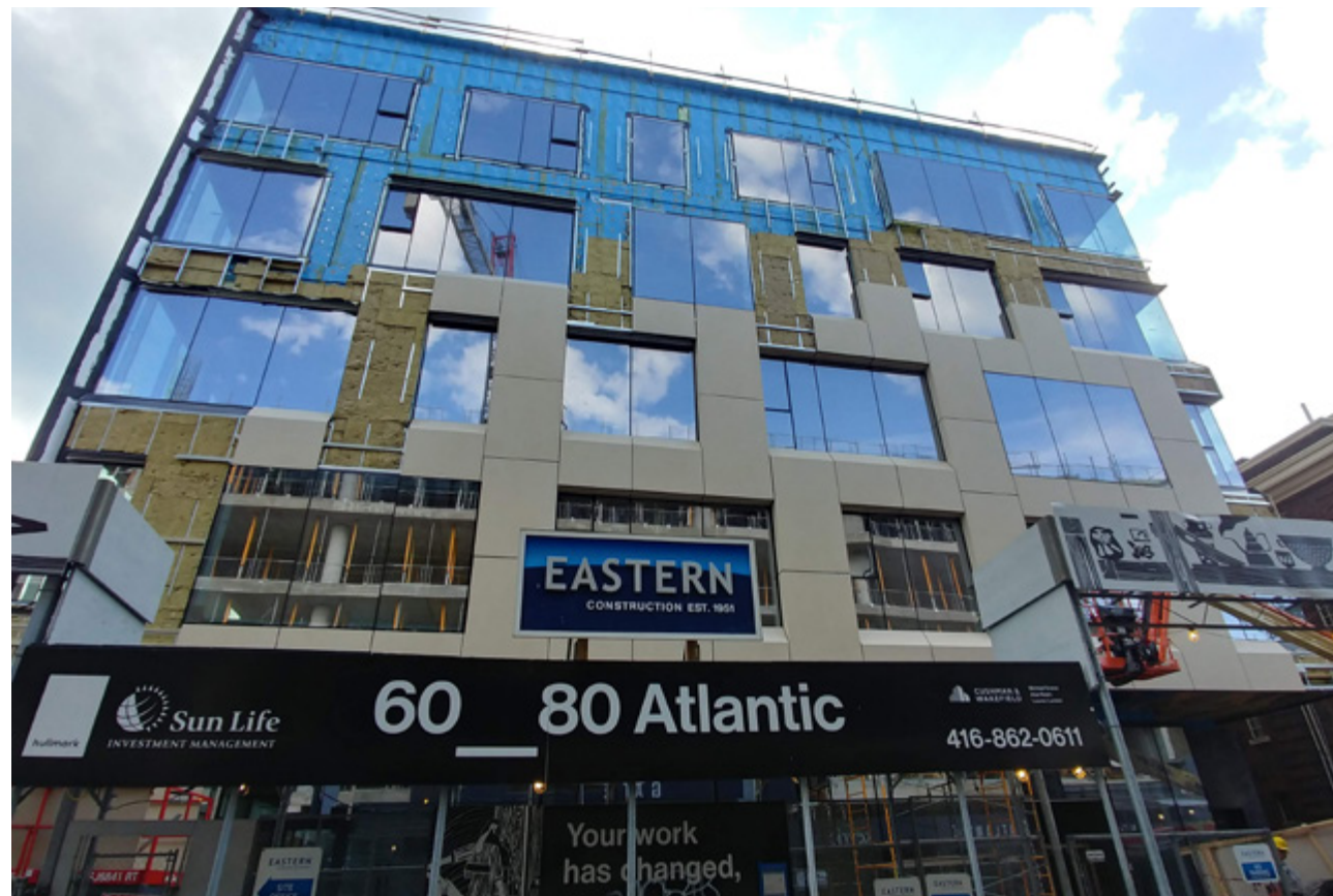
Non-loadbearing steel stud infill framing. Lower floors in reinforced concrete and upper floors in mass timber. A contemporary commercial office façade is rendered over both using conventional components and windows. (80 Atlantic – Julian Mirabelli)
