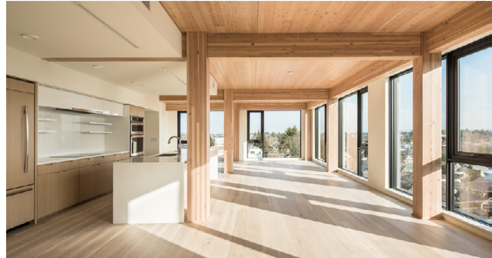
Mass timber post and beam with exposed wood differentiates this innovative project from a typical white-box condo. The Carbon12 mixed-use condominium building in Portland, Oregon employs mass timber, glued laminated timber (glulam) and CLT (cross-laminated timber) in its structural system. (Kaiser + Path)
