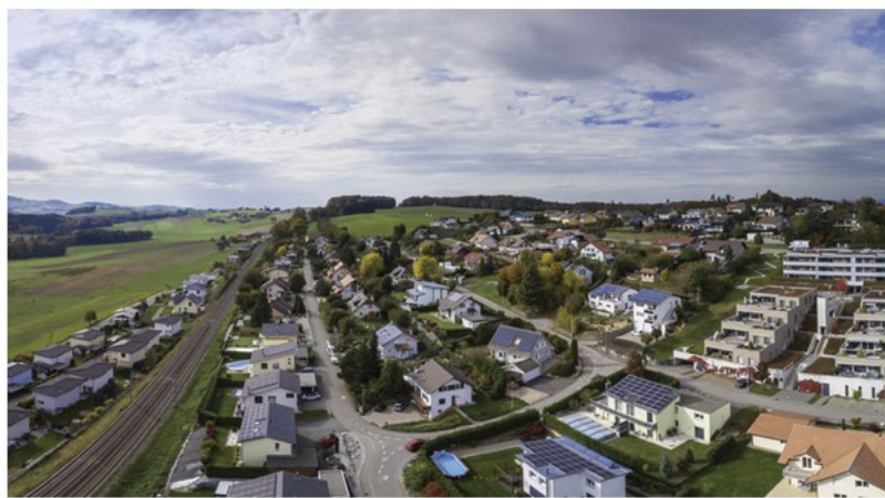
Figure 20: Aerial View of Decentralised Flexibility project site
