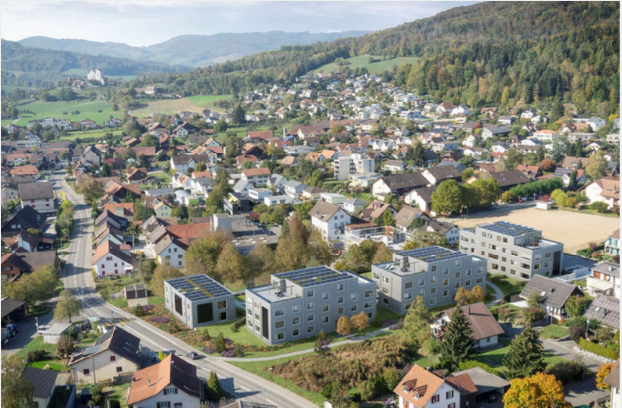
Innovative self-consumption optimisation for multi-family area development with local electricity exchange (page 94 of full report).
