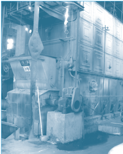
Photos 14, 15 and 16 4-Ton Boilers (14), 6-Ton Boilers (15), and Chilled Water Pumps (16) at the Hubei University of Science and Technology Hospital
