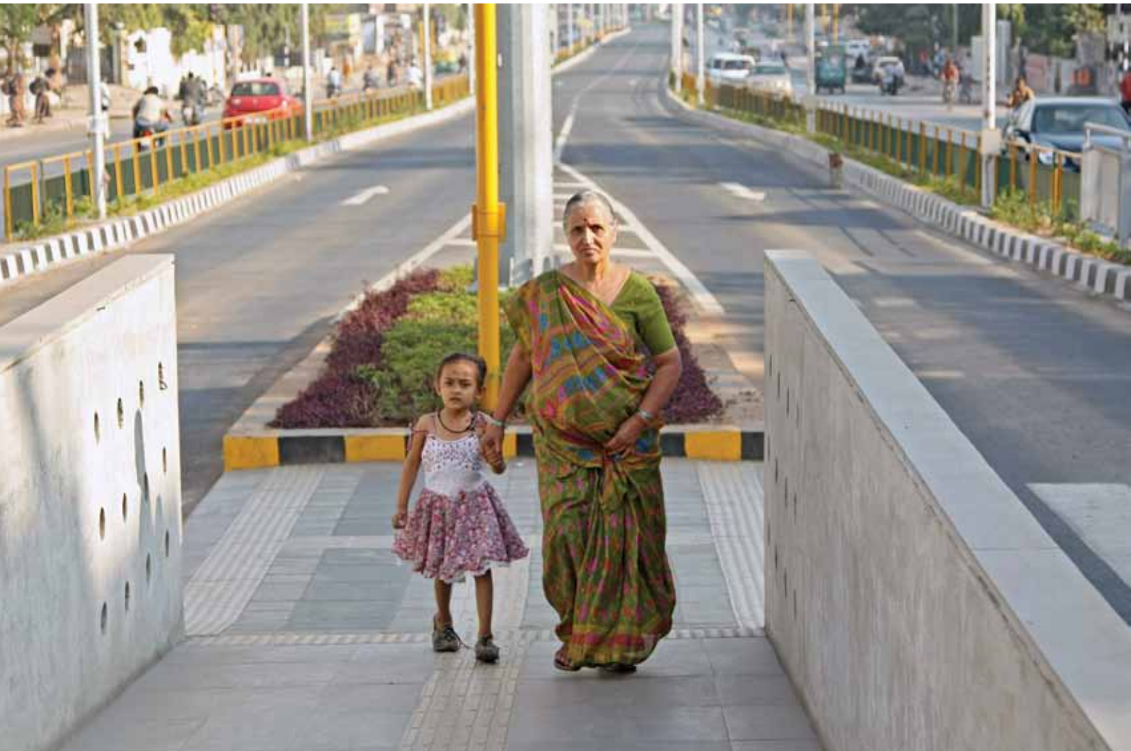
Two Ahmedabad residents enter a new bus rapid transit (BRT) station in a central median. Dedicated high-speed BRT lanes extend behind. Ahmedabad's BRT system, the first in South Asia, focuses on moving people not traffic. Efficiency, affordability, safety, and security are central to the city's transport plan.
