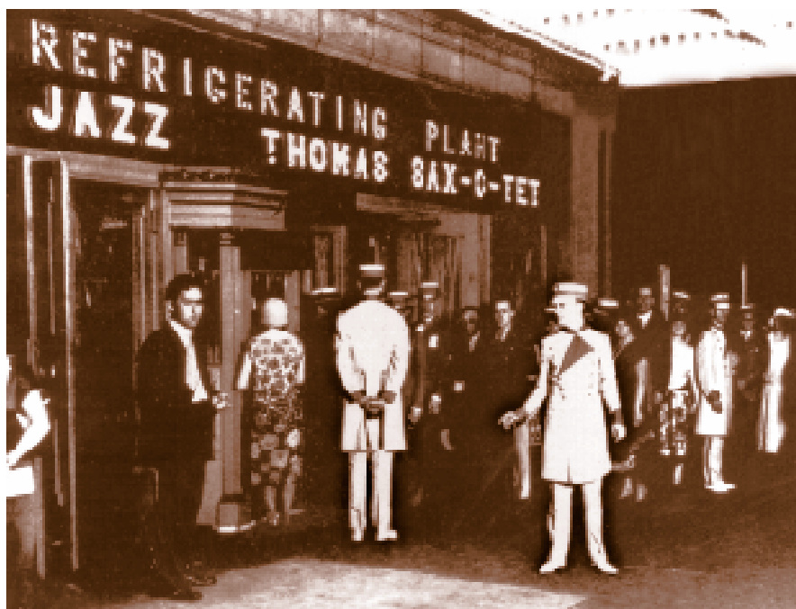
Figure 4: Most Americans’ first exposure to air conditioning was in movie houses and theaters during the 1920s and 30s. Air conditioning was an economic boom to the theater and movie industries.
