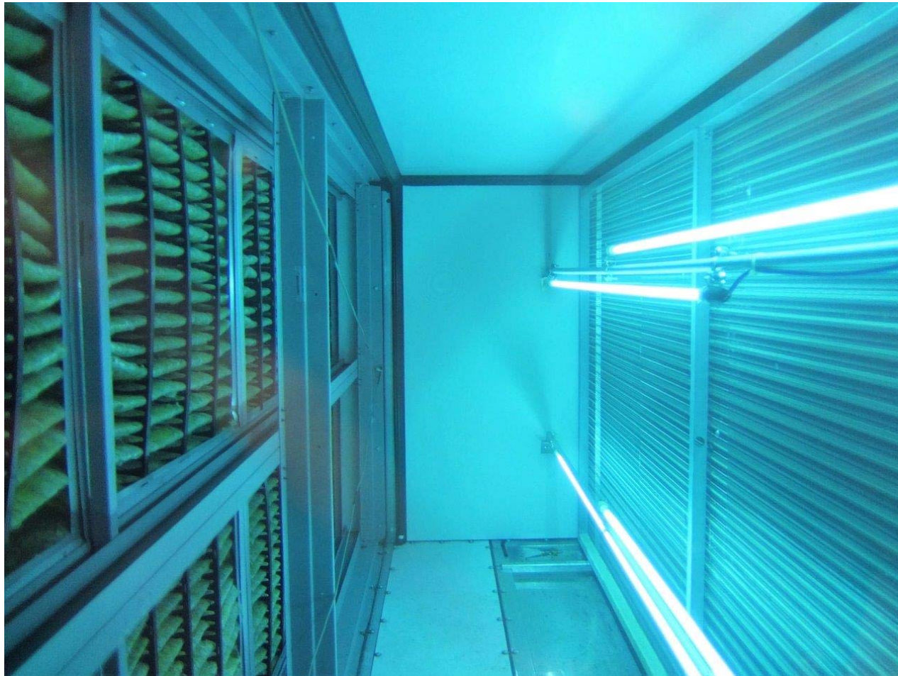
Downstream coil surface/air installation
