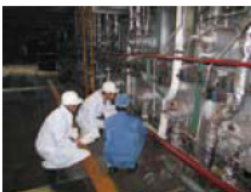
Audit of thermal insulation and heat retention of a factory furnace
