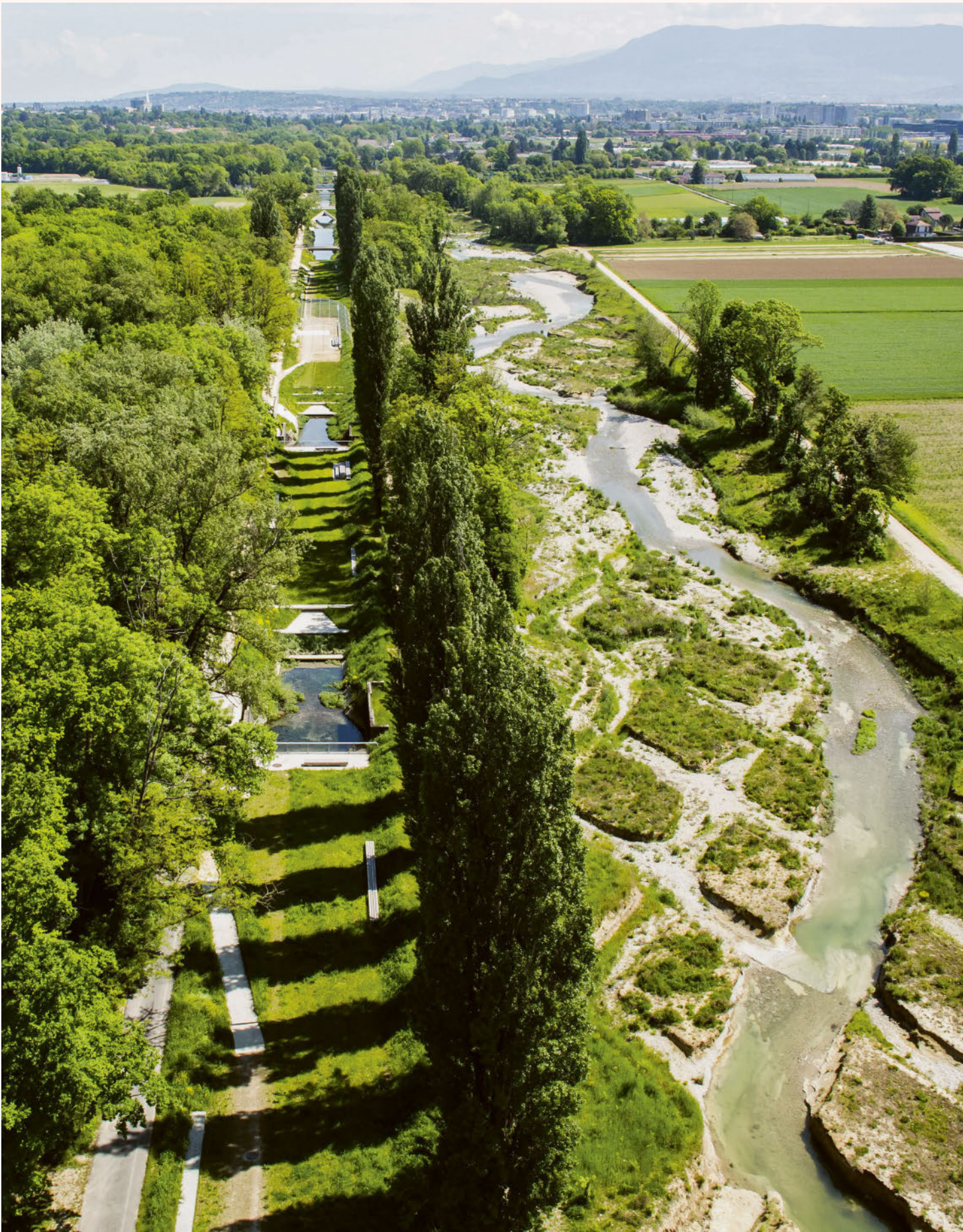
Following the rehabilitation of the small River Aire in the canton of Geneva, the river is able to wend its own way through diamond-shaped dredged furrows.
