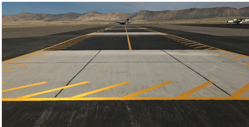
Figure 3-1. Rehabilitated Surface of Cal Pad W5
