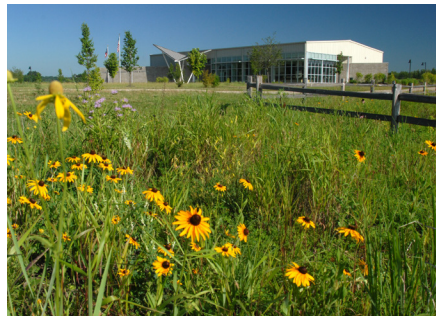
Fernald Preserve Visitors Center, Ohio
