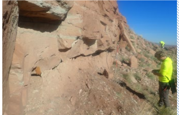
LMSP DRUM Field Team Lead Zack Schuler records data for a closed (backfilled) adit at the Chester Mud 1 mine in Arizona.
