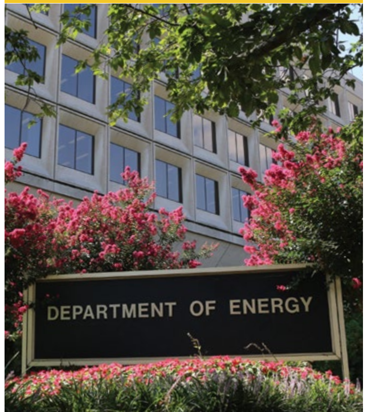
James V. Forrestal Building, Washington, D.C.
