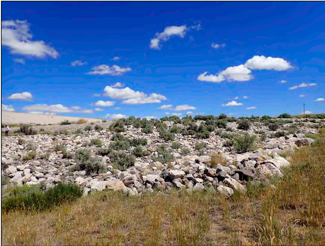
PL-13. Diversion Channel No. 2
