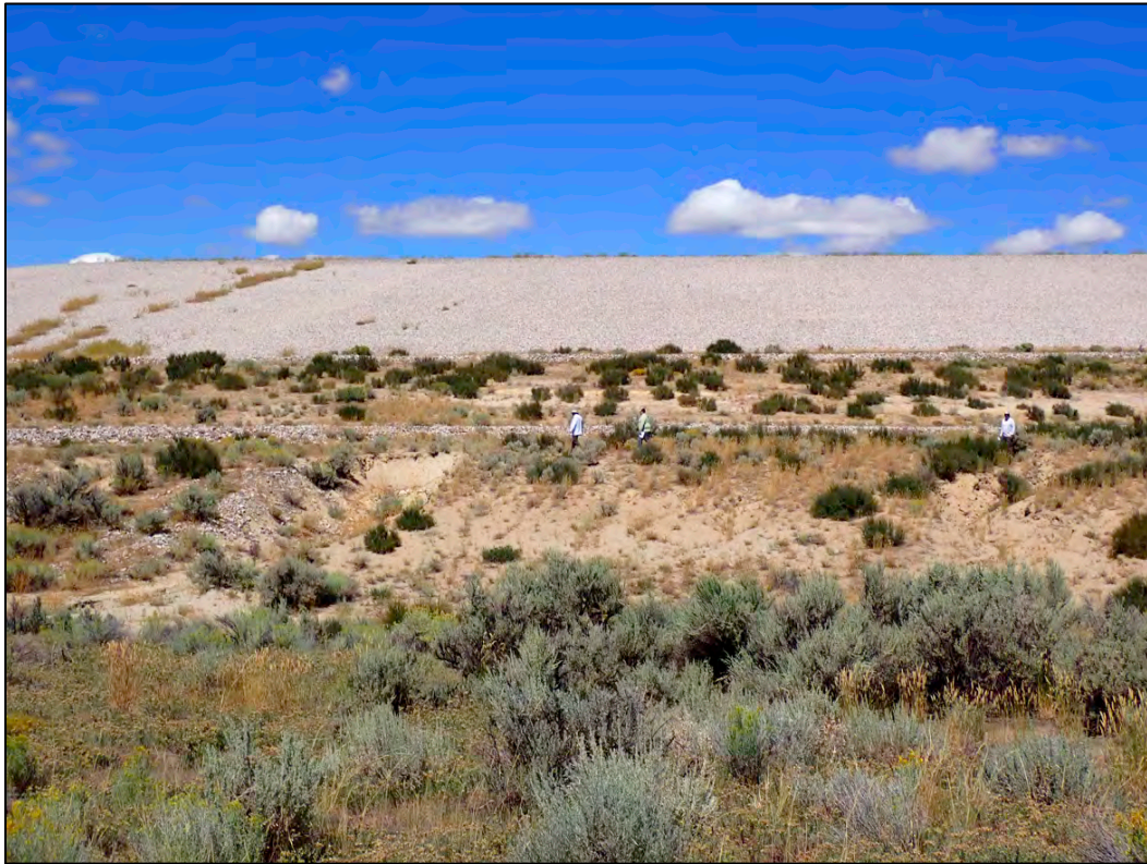
PL-15. Erosion Below Rock Berm
