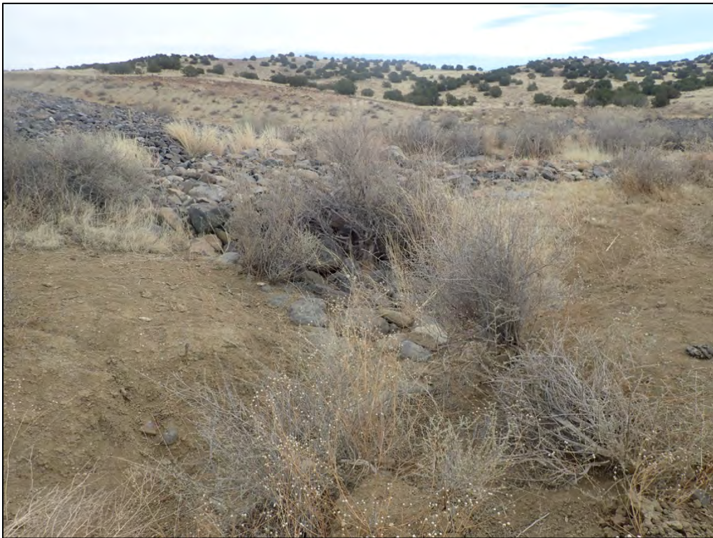
PL-20. Rilling Contacting South Channel Cutoff Wall
