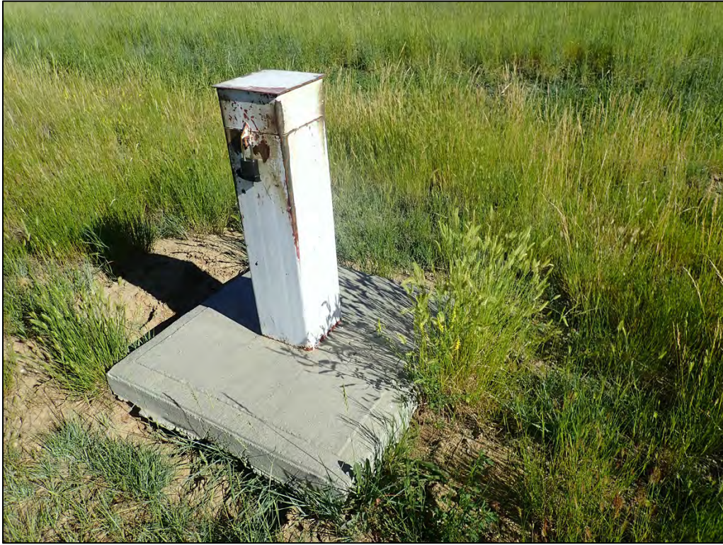
PL-5. Burrowing Near Monitoring Well 40-SC
