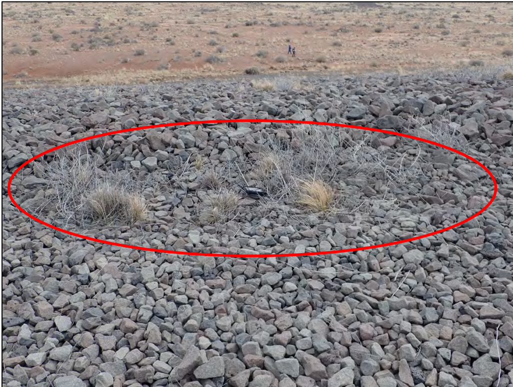
PL-13. Potential Depression Area on Top Slope at Top Slope/Side Slope Boundary
