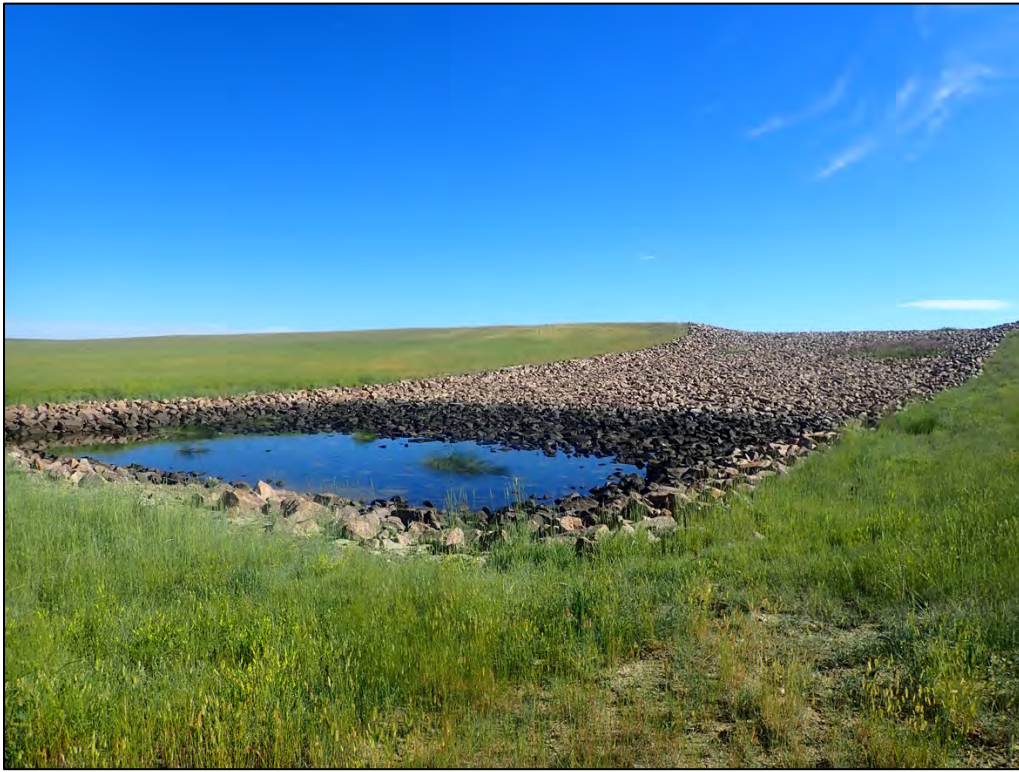
PL-11. South Swale Discharge Point
