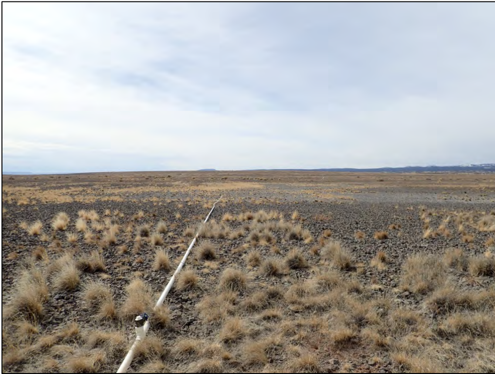
PL-11. Overview of Siphon and Vegetation on Disposal Cell Top Slope
