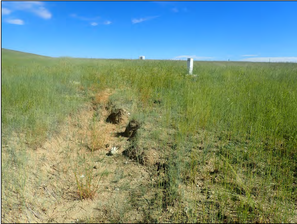
PL-14. Erosion Caused from Overflowing Water Storage Tank
