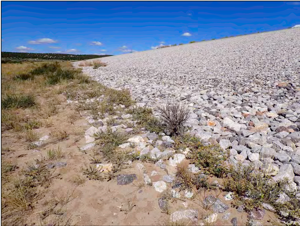
PL-7. Windblown Sediment Accumulation at Toe of Side Slope
