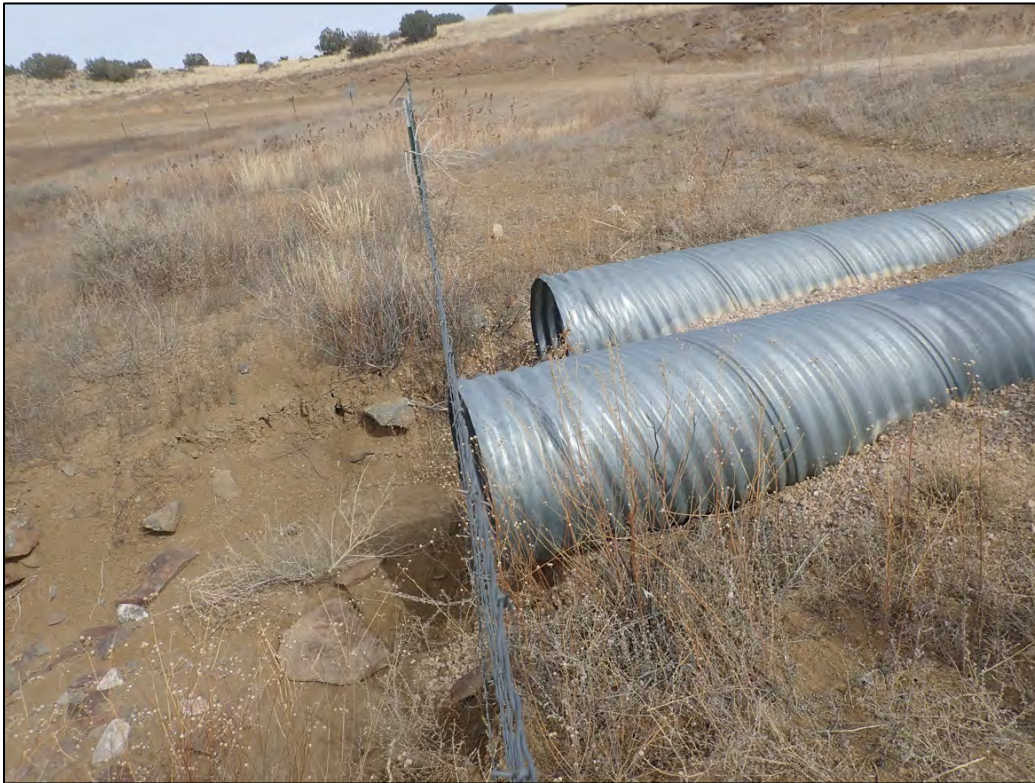
PL-1. Culvert Outlets Along Access Road near Perimeter Sign P9
