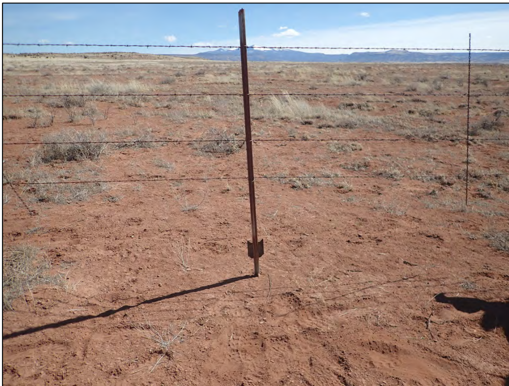
PL-2. Wind Erosion on Eastern Fence Line (Hanging T-Post)
