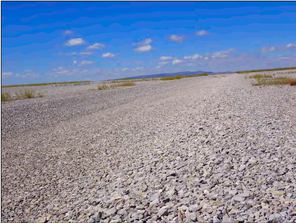
PL-11. Diversion Channel No. 1
