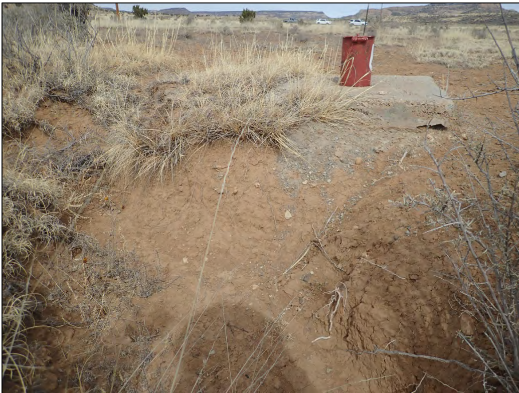
PL-8. Erosive Channeling Around Monitoring Well 62
