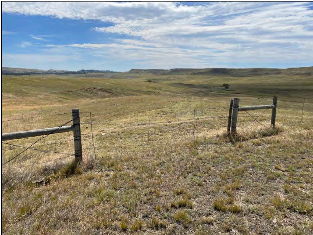
PL-2. Southeastern Side Perimeter Fence Gate
