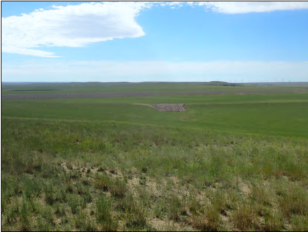
PL-6. Overview North Side of Disposal Cell and North Swale Discharge Point
