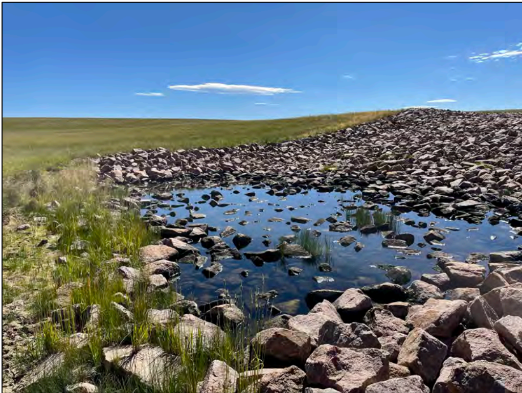
PL-10. North Swale Discharge Point
