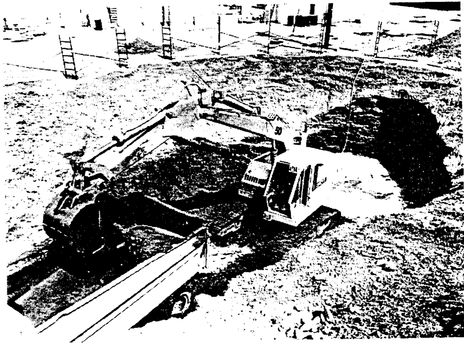
Figure 5. Site Excavation--Advanced Stage
