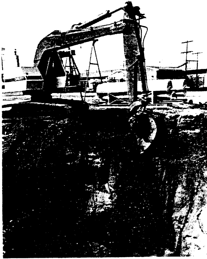
Figure 4. Site Excavation-- Initial Stage
