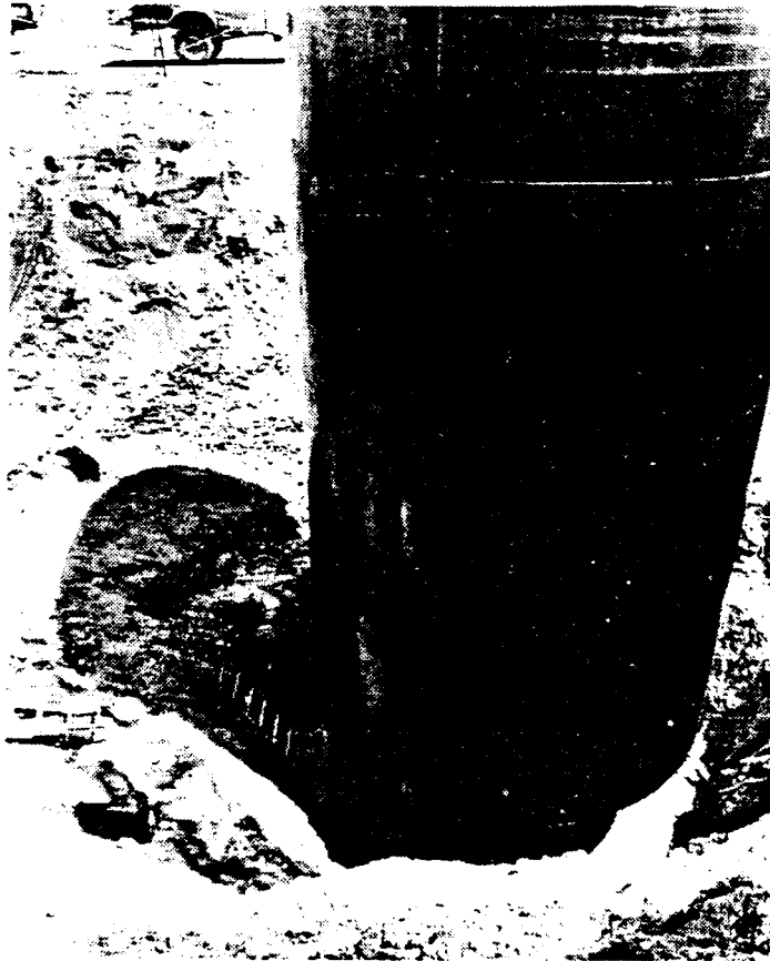
Figure 8. Steel Shell Emplacement
