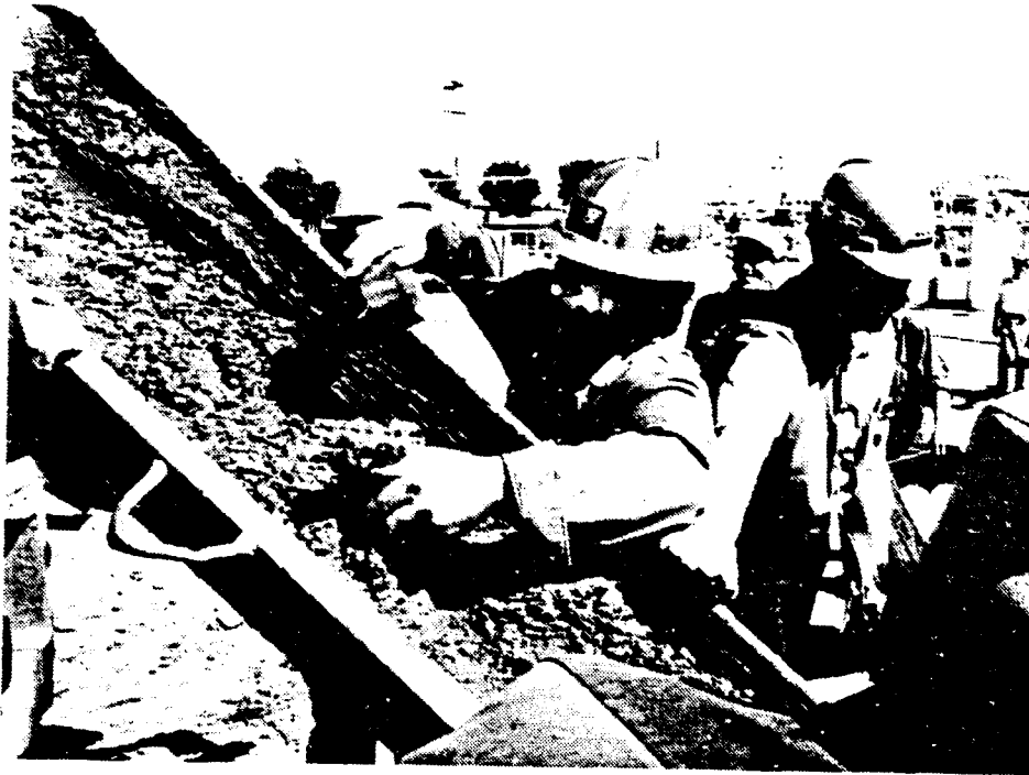
Figure 13. Collecting Samples of Concrete Mix
