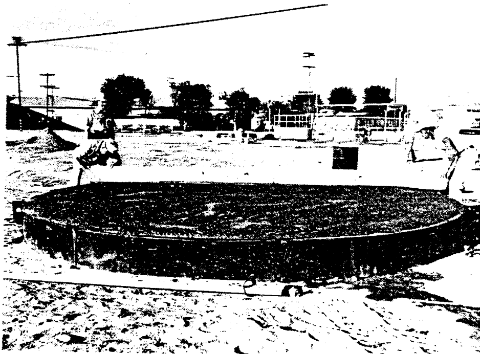
Figure 14. Leveling the Concrete Surface
