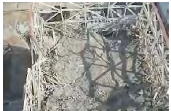
Figure 9: View of Unit 1 after the hydrogen explosion; source TEPCO
