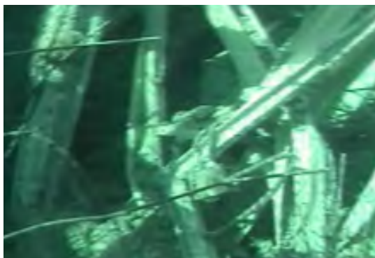
Figure 13: Debris in the spent fuel pool, Unit 3; source Ref.18
