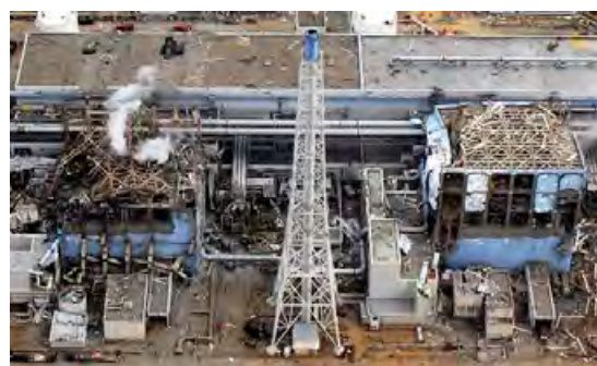
Figure 14: Units 3 and 4 after the hydrogen explosion; source: TEPCO
