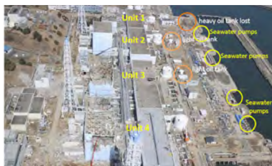
Figure 6: Failure of cooling water supplies (Dai-ichi); source: University of Japan
