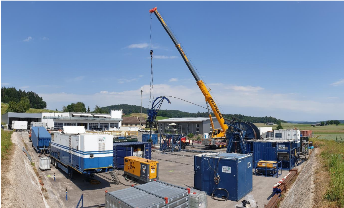
Figure 9: Backfill operations of Nagra's deep drilling site "Stadel-2" in 2023 (Photo ENSI).
