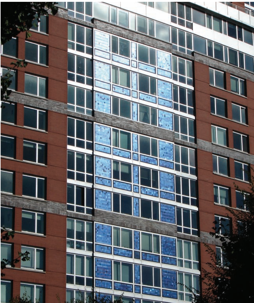
The Solaire features 3,400 ft 2 of custom-laminated and standard photovoltaic modules.
