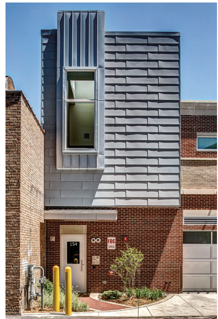
Rear entrance. The brick pavers and concrete driveway are each protected from snow and ice with a melting system using a weather predictive demand-control activation algorithm.
