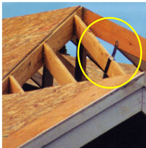
Figure 6 - A bolt-on anchor attached to a rafter.
