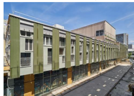
FIGURE 6: SHOT OF THE SOUTH WALL OF THE BUILDING ELYS
