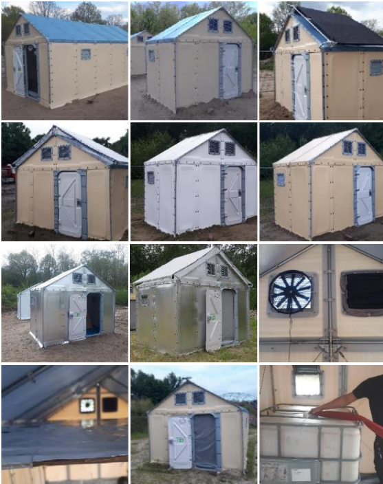
Fig. 2: In reading direction: Standard full shelter, standard one-third shelter, one-third shelters with black shade net, aluminum shade net, white paint-coated envelope, grey foam panels and beige paint-coated roof, aluminum-coated envelope, and aluminum-coated envelope with aluminum shade net, Exhaust fan applied to vent in the full shelter, Interior ceiling under construction in the full shelter with the exhaust fan in the background, additional door for cross ventilation in the full shelter, water tank for thermal mass in the small shelter
