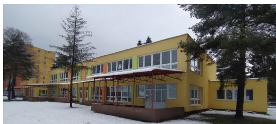
Figure 1 External view on the south-east side (rear entrances)
