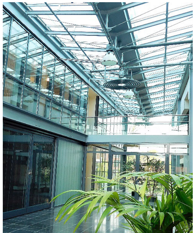
Figure 1. The Gemeentehuis Horst building.
